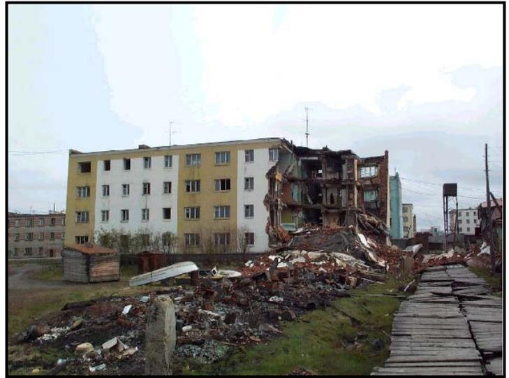
Four-story apartment building in Cherski, North-East Yakutia (upper Kolyma River) was destroyed because of permafrost thawing and differential settlement in its foundation. It took only several days between the appearance of first cracks in the walls and the partial collapse of the building. Photo by Prof. Vladimir Romanovsky, University of Alaska Fairbanks.
