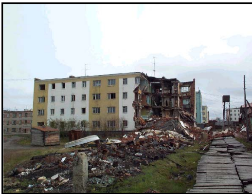
Four-story apartment building (not public infrastructure) in Cherski, Russia, North-East Yakutia (upper Kolyma River) was destroyed because of permafrost thawing and differential settlement in its foundation. It took only several days between the appearance of first cracks in the walls and the partial collapse of the building. Photo by Prof. Vladimir Romanovsky, University of Alaska Fairbanks.
