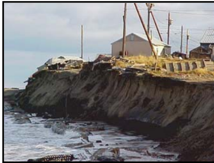
Bluff erosion & permafrost thaw, Shishmaref (c 2002) Kawerak
